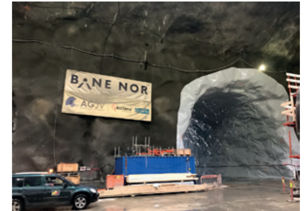
AGJV BANENOR OSLO - FOLLO LINE PROJECT
